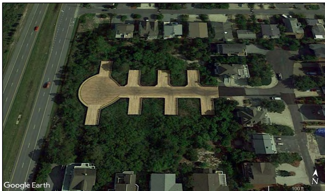
Figure 4. Google Earth image showing the constructed elevated driveways for future houses in the Tower Shores development.
